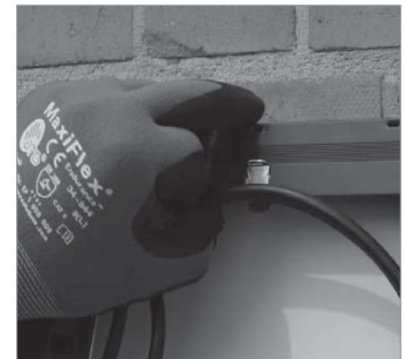
**PRE-INSTALL MLPE:** Install MLPE in a location on the module that will not interfere with microrails or grounding lugs. To use trunk cable most efficiently, install MLPE components in the same locations on all modules in the same row.
